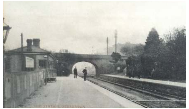
Figure 30: The former station buildings have since been demolished
