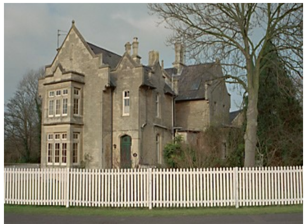
Figure 33: Grade II Listed Station House & The Sycamores
