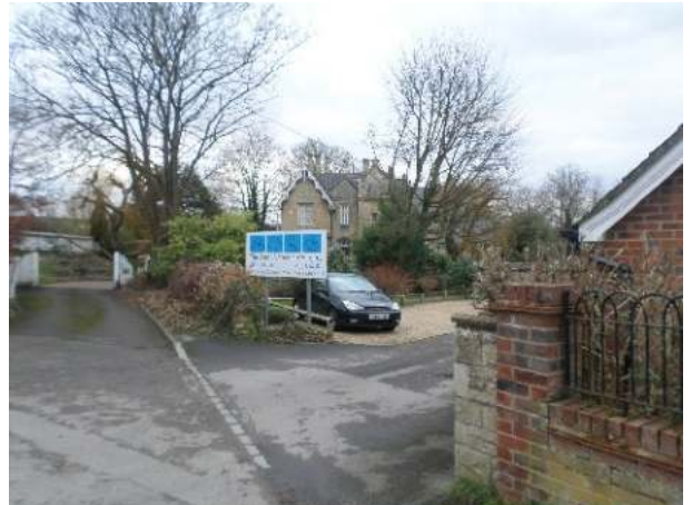
Figure 31: View across the Veterinary Surgery entrance to the historic station buildings
