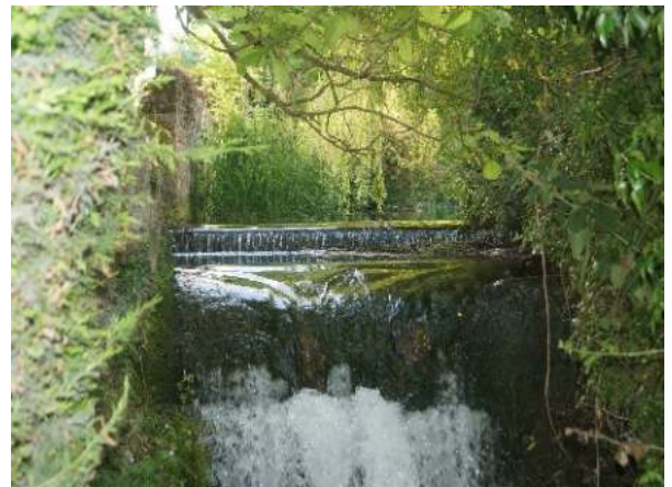
Figure 43: Mill Street stream
