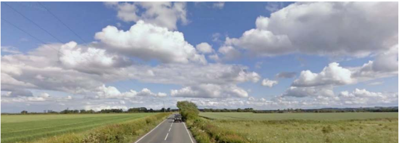
Figure 80: View along Hanney Road
