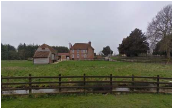
Figure 42: Grade II Listed Manor Farm and Granary
