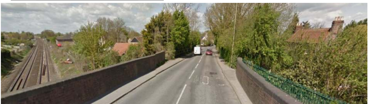
Figure 37: View westward along the railway line
