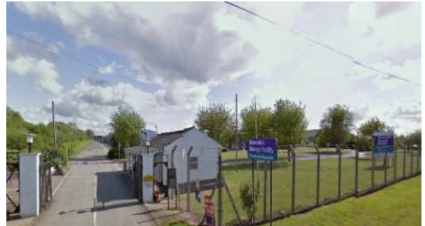
Figure 79: Storage Depot Entrance
