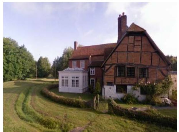
Figure 40: Old Farm House
