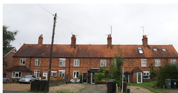
Figure 57: Victorian terrace built to house workers for Robert Langford
