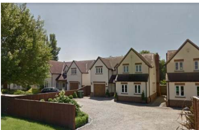
Figure 75: 91 -97 Hanney Road - comprises 4 detached brick and render dwellings. Reflecting the materials of adjacent properties, respects the existing building line and the well landscaped surroundings
