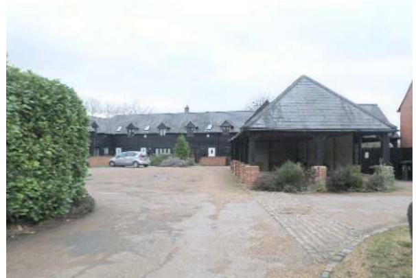
Figure 76: Timsbury Court - this courtyard development successfully introduces a relatively dense form of development, but retains the rural appearance of the many agricultural buildings in the settlement.
