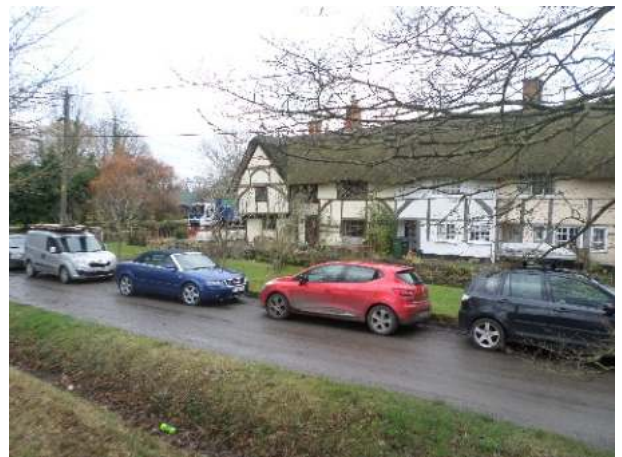
Figure 25: Timber framed housing on Milton Road - with on-street parking detracting from the street scene
